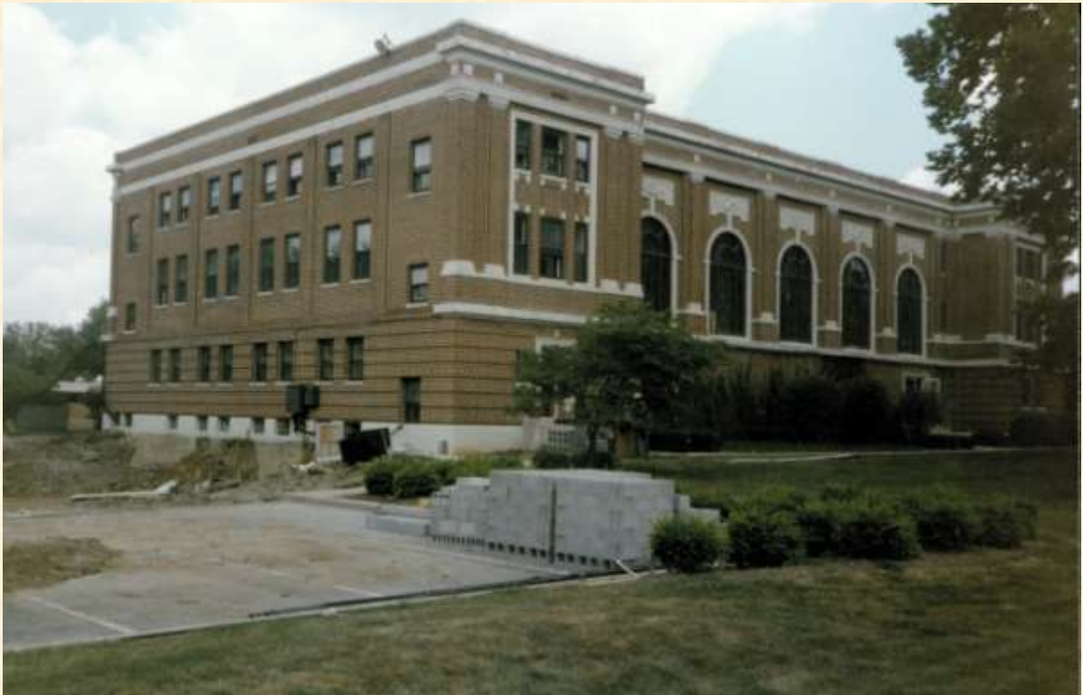
West Side of Presser Before Practice Room Addition
