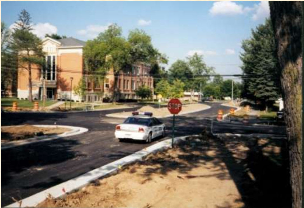
Looking East Along College Ave.
