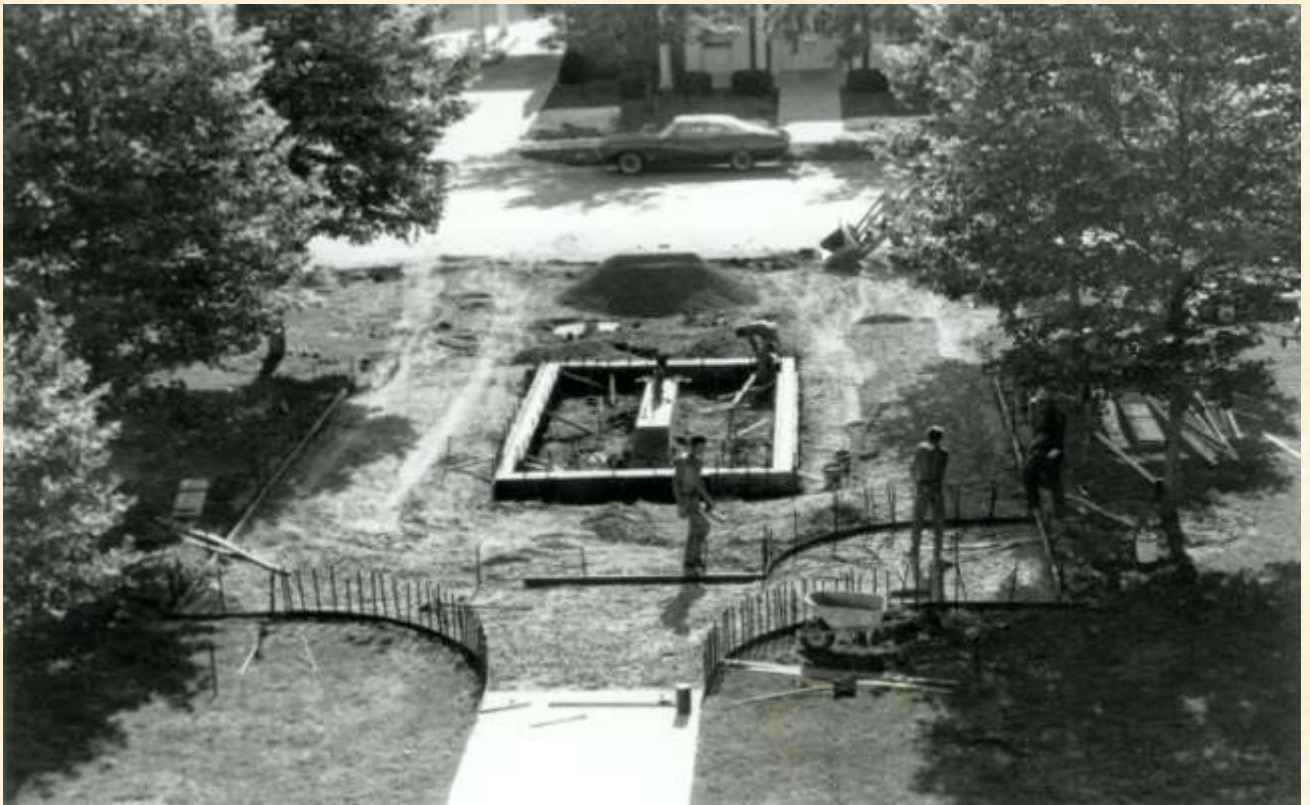
View of Plaza Construction From Lehr Memorial
