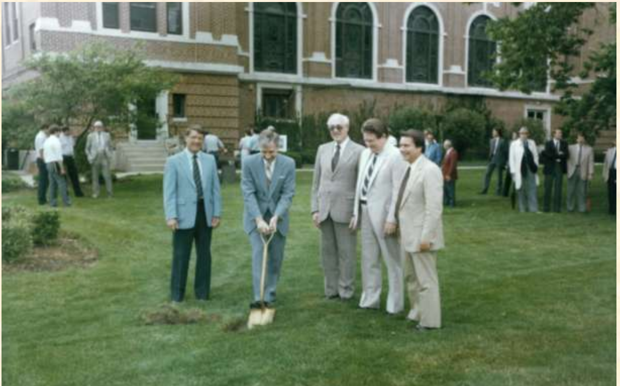
Groundbreaking For Presser Hall Renovation President Freed With Shovel
