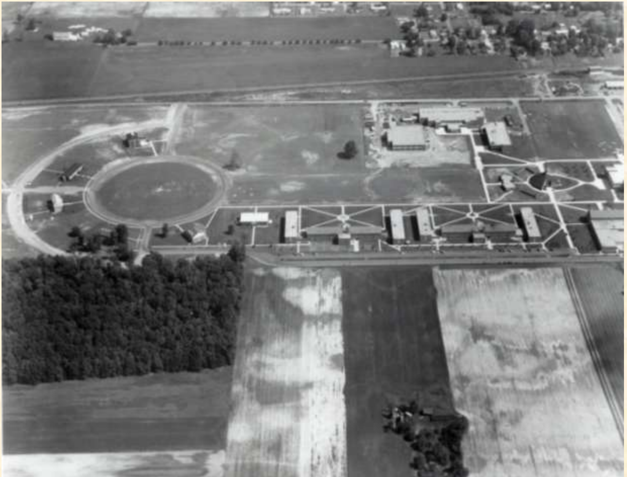
West Campus in Early 1970's Upper Right – Pharmacy and Meyer Hall Completed Biggs Engineering Building Under Construction Looking North
