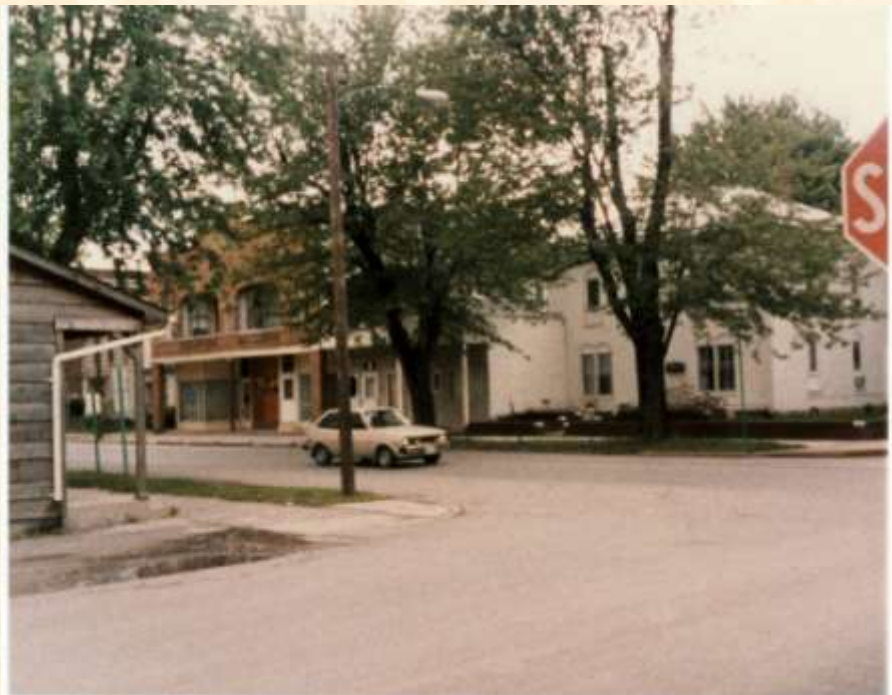
View from Corner of S. Main St. and Lehr Ave. – Looking South
