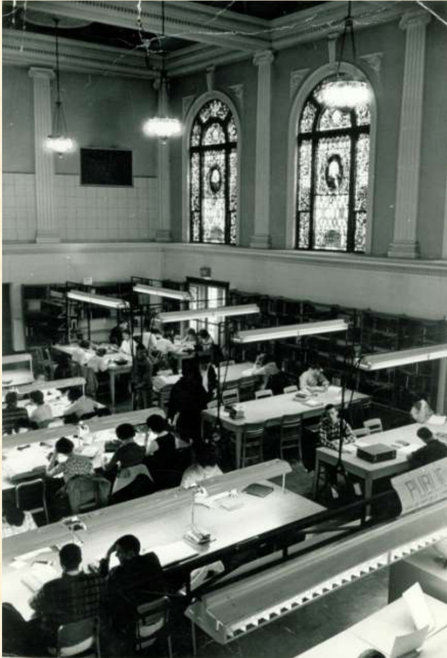
Former Willis Auditorium Converted to Reading Room Currently (2008) Snyder Recital Hall
