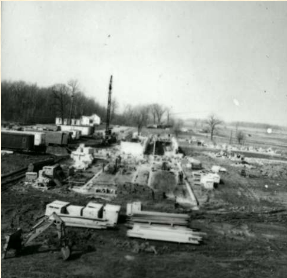
Lima Hall Under Construction – Looking West
