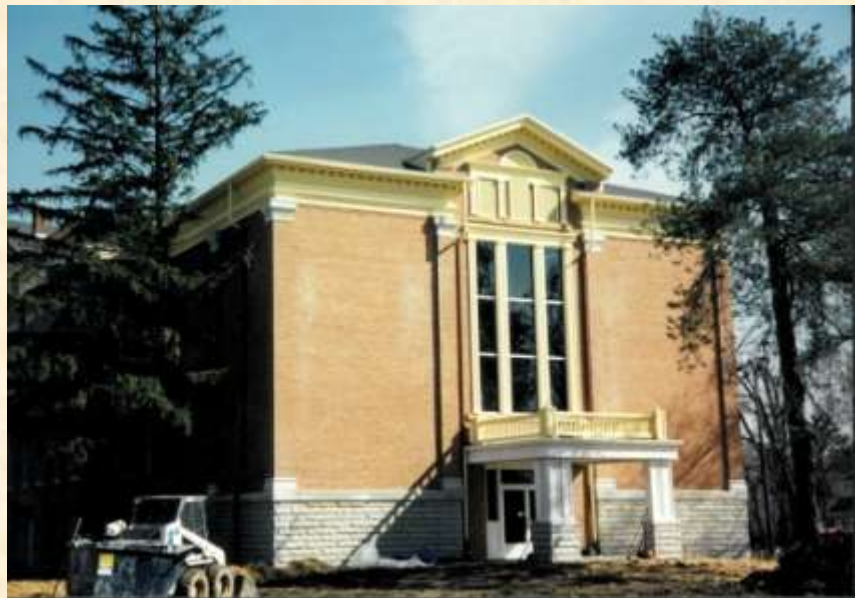
West End of Freeman Annex
