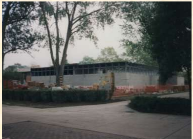
Same Area with Construction Underway
