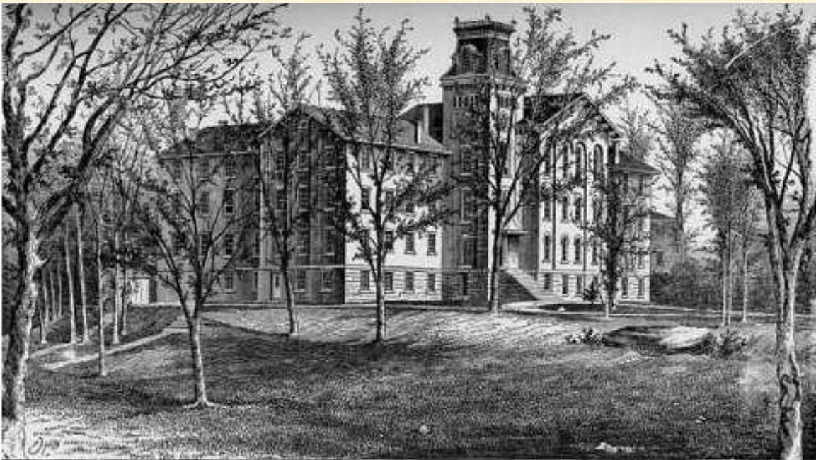
MONNETT HALL, OHIO WESLEYAN UNIVERSITY, DELAWARE, OHIO (ORIGINAL BUILDING)
