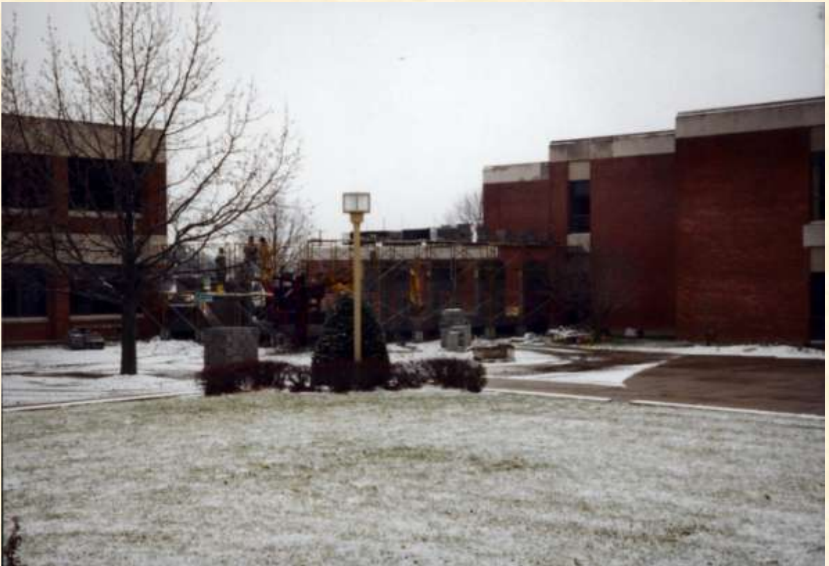
Meyer-Biggs Annex at Start of Construction
