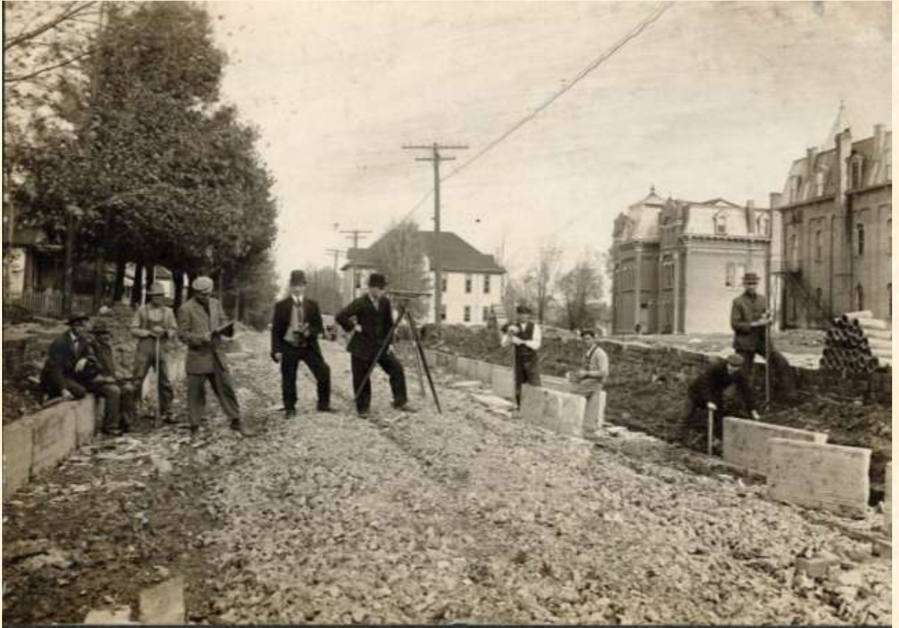
Paving South Gilbert Street – (R to L) Normal School Building, Administration Building Pharmacy Building in New Location Between 1909 and 1913
