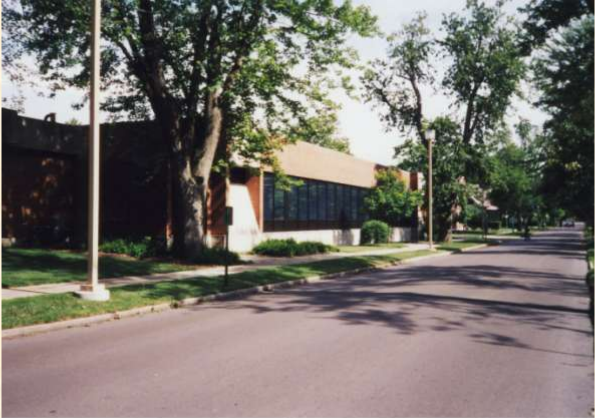
Completed Hanson Annex from S. Gilbert St.
