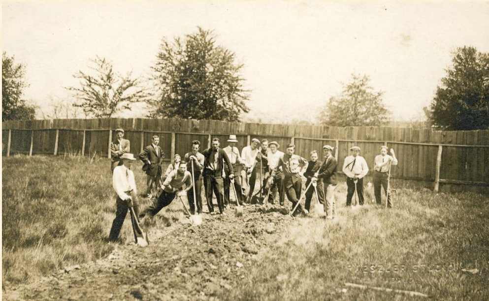
Early Civil Engineering Students Grading a Drainage Ditch
