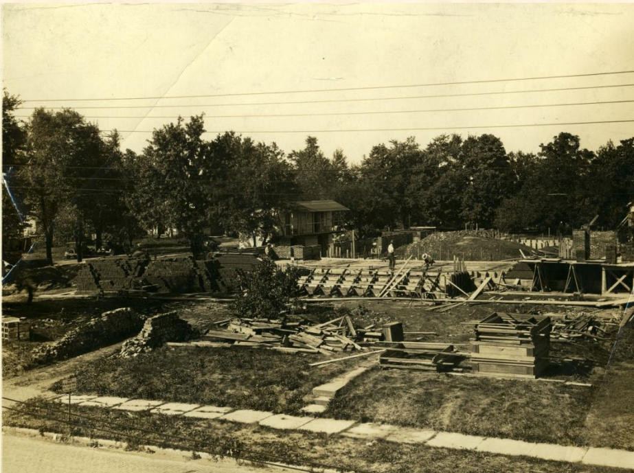
Presser Hall Under Construction
