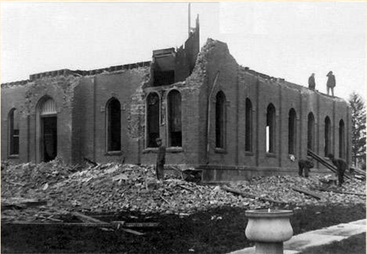
Demolition of Normal School Building In Preparation for Lehr Memorial
