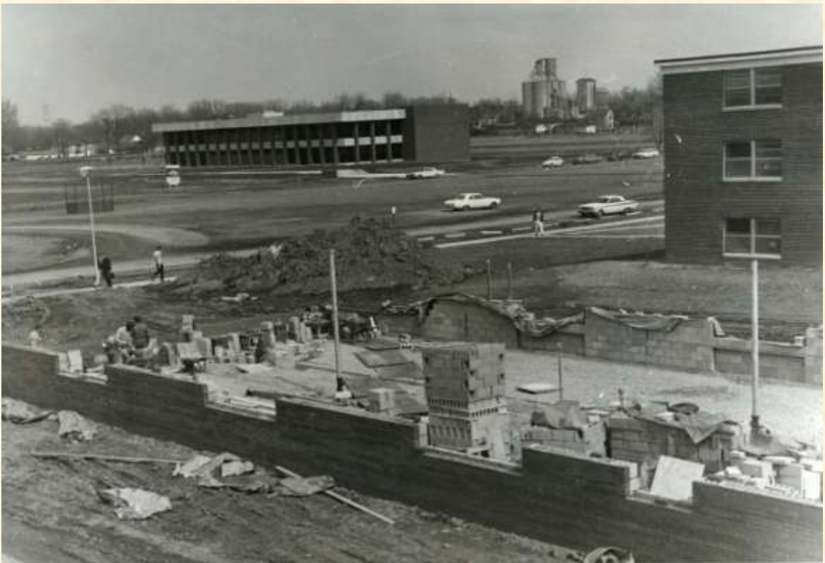
Construction of Park Hall Pharmacy Building in Background
